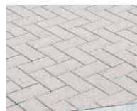
Keyblock paving
