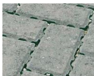
Permeable keyblock paving
