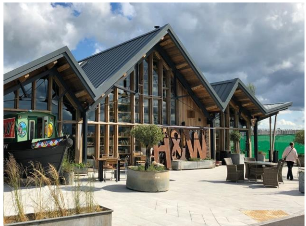
Division of the roof into a number of smaller elements and expressed gable ends creates interest and variety.
