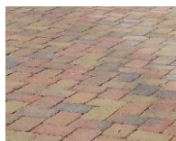
Concrete setts / block paving
